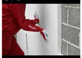
Foam adhesive with EasyGun applicator for fixing and sealing rigid insulation boards
