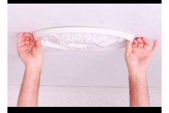
Acrylic adhesive for installing interior polystyrene decorative elements and boards
