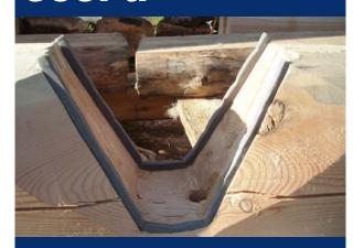
Self-expanding elastic tape for sealing connection and expansion ioints
