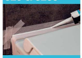
Acetoxy sanitary silicone for sealing works in wet and humid areas
