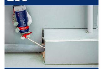
Filling straw foam with pest- and mice-repellent additives
