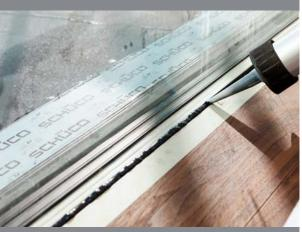
Hybrid sealant for filling and sealing high movement connecting joints
