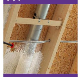
Sprayable gun foam for thermal and sound insulation
