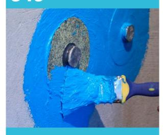
Fibre-reinforced waterproofing mastic for wet and humid areas
