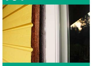
Elastic seamless liquid membrane for sealing external window and door joints
