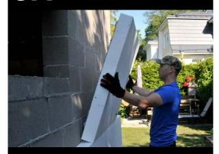
Foam adhesive for fixing exterior and interior insulation boards
