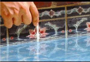
Two-component fast-curing epoxy putty for quick repair works on damp, wet and underwater surfaces
