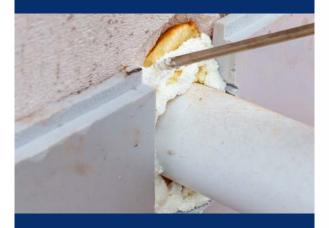
Multipurpose construction gun foam for various sealing and filling works
