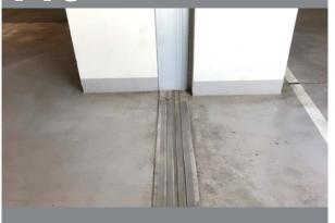
Self-levelling hybrid sealant for heavy-wear horizontal floor joints
