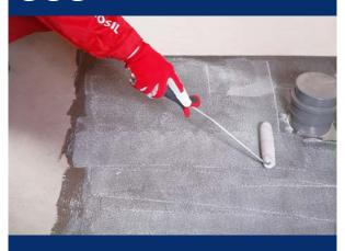
Water-based primer that strengthens and improves adhesion and primes interior and exterior surfaces prior to finishing works
