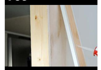
Elastic hybrid adhesive and sealant for moveable joints (±12.5%)
