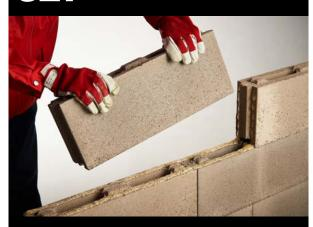
Adhesive gun foam for fastening construction blocks and stones in non-load-bearing interior walls
