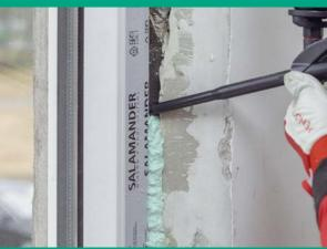
Elastic gun foam for window and door installation
