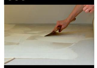
Acrylic adhesive for gluing various soft floor- and wall-covering materials
