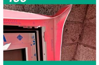
Double-sided window tape for moisture and air proofing internal window and door joints
