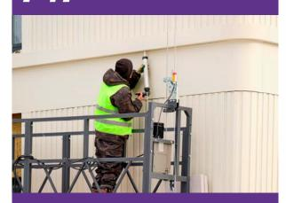
Elastic MS polymer-based hybrid sealant for sealing various facade joints
