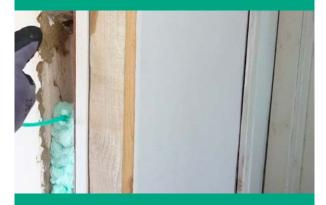
Elastic straw foam for window and door installation
