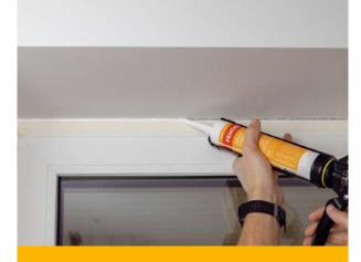
Paintable elastic sealant for filling moveable (±12.5%) gaps and joints
