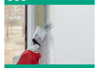
Fibre-reinforced vapour-proof mastic for sealing internal window and door **joints**
