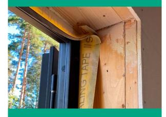
Moisture barrier tape for internal window and door joints
